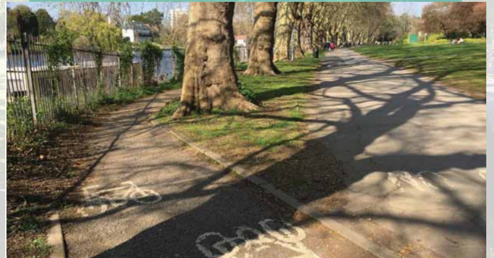
Top: Existing cycle path Bottom: Entrance southern end
