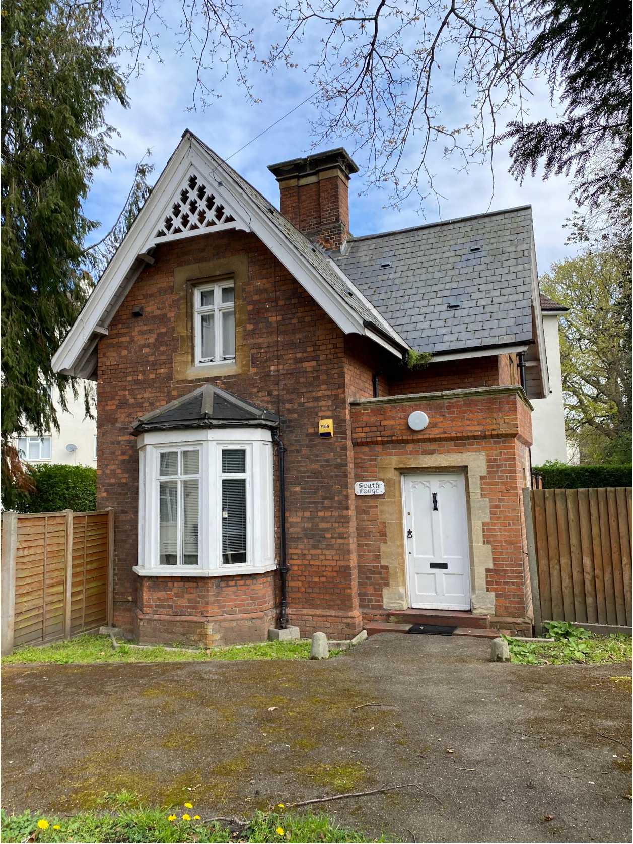
Front (northwest) elevation
