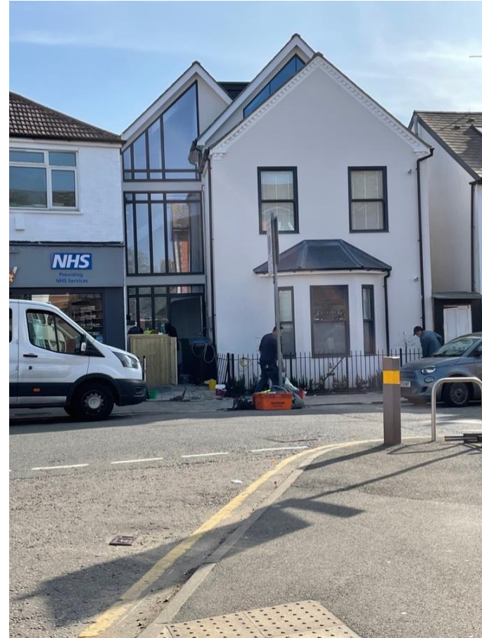
Renovated and reconfigured as homes in 2022 Note the successful piggyback approach to additional roof storey and contrasting and entirely modern approach to the glazing of the new additions.
