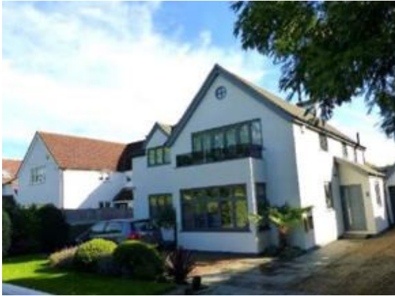
Lower Ham Road: Modern additions
