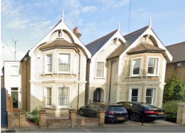
Park Road: Considerate 3 storey side extension enhancing the property overall
