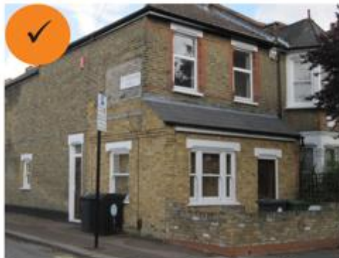
Corner conversions should provide windows on both street elevations where possible
