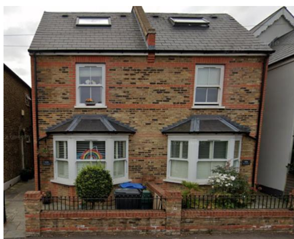
Elm Road new infill housing
